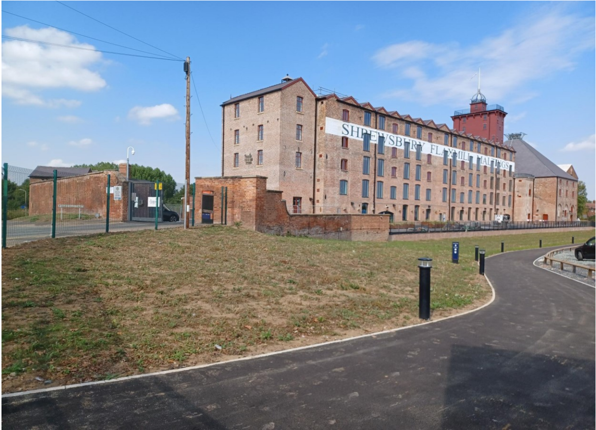
- Shrewsbury Flaxmill Maltings, from the junction of Crewe Street and St Michael's Street –
